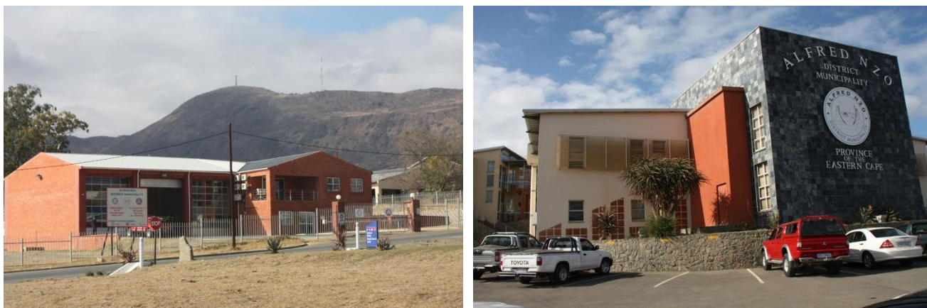
Figure 1 District Disaster Management / Fire Services Centre (left) and the District Municipal offices (right) in Mount Ayliff
